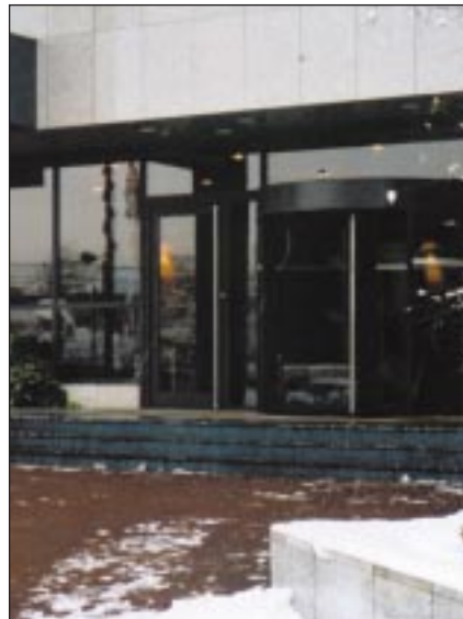
Snow and ice prevention at building entrance
