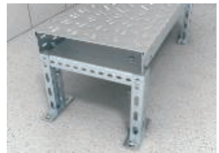
Installation and fastening of the walkable cable tray system for floor stand-off.
