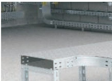
Walkable cable tray system, stand off on U profile structure.
