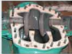
Reclaiming totally eroded surface
