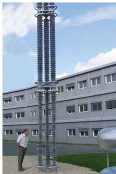
Station Post for 800 kV DC
