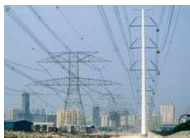
DEWA's 420 kV Compact Line
