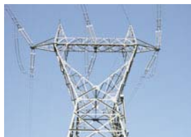
ATEL's 420 kV Line with 500 kN Force Rating
