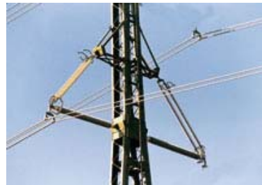
420 kV Braced Line Post erected in 1998
