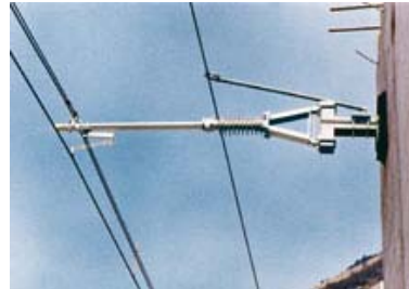
Catenary Installation for the Swiss Railway installed in 1979
