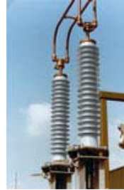
123 kV Cable Termination installed in 1975
