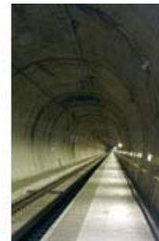
High Speed Track in the Swiss Loetschberg Tunnel
