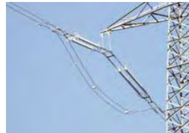
420 kV Suspended Double Tension Set
