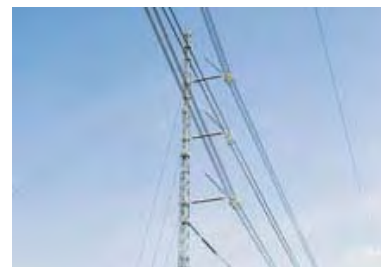
420 kV Suspended Double Tension Set
