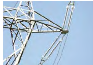
420 kV Double Tension Set
