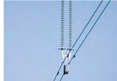
420 kV Double Suspension Set
