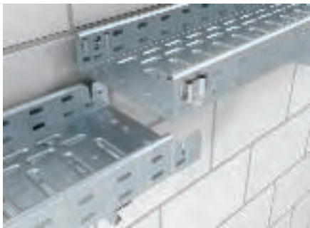
Straight connection, cable tray interconnection
