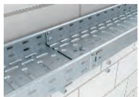
Connection of the cut end with the interconnection end
