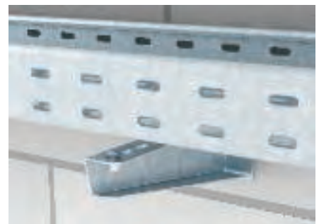
Standard cable tray mounting on the wall with wall and support brackets.
