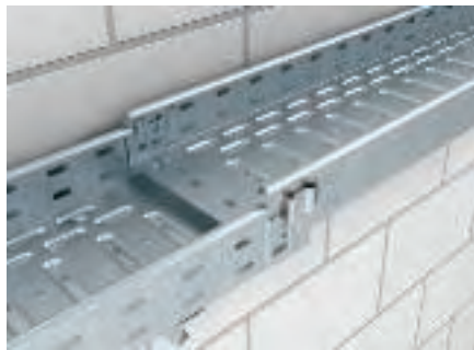
Straight connection, cable tray interconnection
