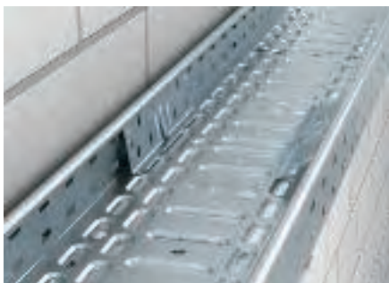
Installation of RV connector set
