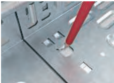
Straight connection, cable tray interconnection
