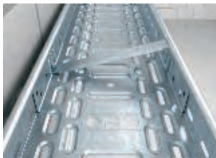
Installation of RV connector set
