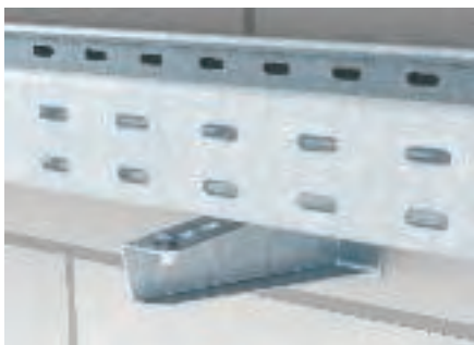
Quick fastening of cable tray on the bracket
