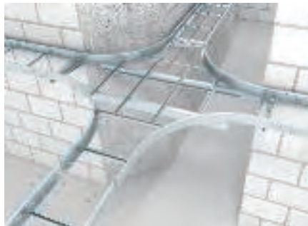
Installation of an cross-over, type LK, for the creation of two exits. Additional supports should be planned for the area of the fittings.
