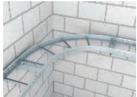
Connection of the cable ladder with the bend, type LBI 90. Additional supports should be planned for the area of the fittings.
