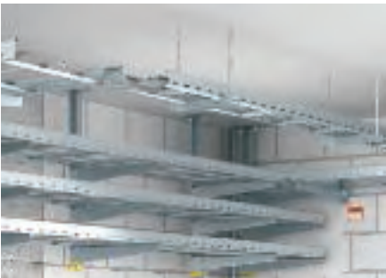
Example of installing cable ladders with supports of U profiles and threaded rod suspension.
